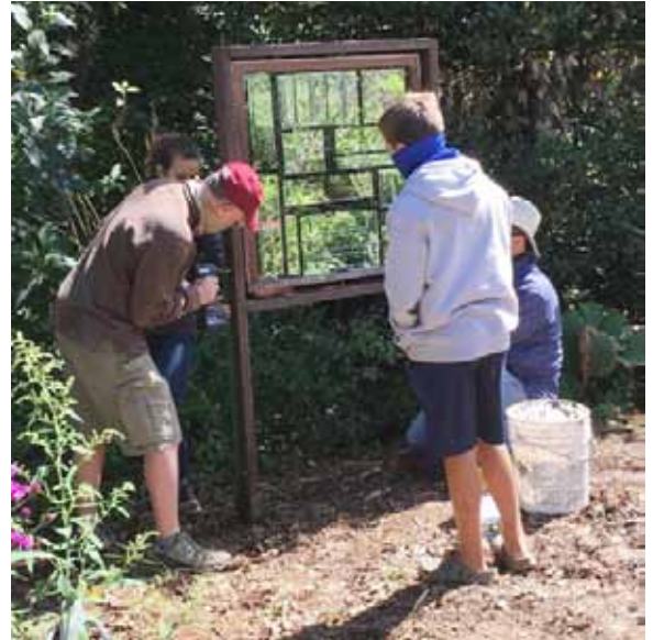
Dave Angle, left, at work installing a public art project.
